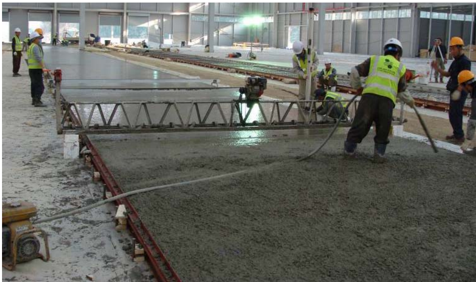
Figure 10: Long strip construction
